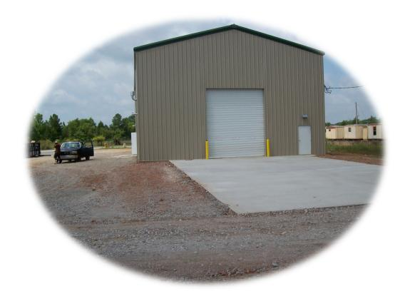
**Project B** – G & M Associates provided and constructed a 20 ft. x 40 ft. x 18 ft. pre-engineered metal building for use as a parts storage warehouse at the Combined Surface Maintenance Storage Building in Smyrna, Tennessee. The building was constructed of a pre-engineered metal building structure including all systems and new utility services. Construction was done on federal land, and met International Building Code and all other applicable building codes.
